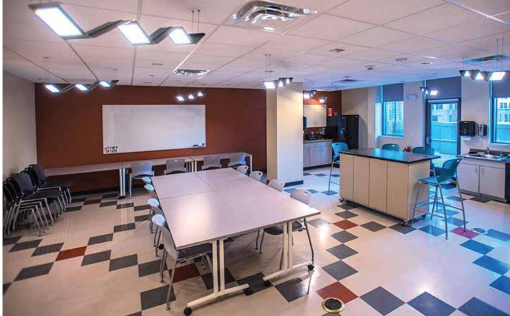
OLED Gateway program installation at DeJoy, Knauf & Blood office, in Rochester, N.Y.
