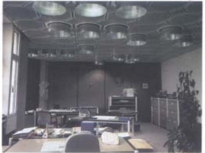
The lighting fixtures are out of proportion and 'threatening' rather than pleasant. The nature of the material and the brightness of the ceiling are inappropriate.
