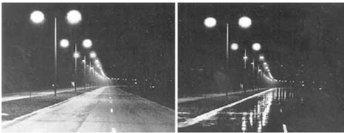
Fig. 5 Different Visual Impressions of the Road Surface Under the Same Lighting Level for Dry (Left) and Wet (Right) Conditions
